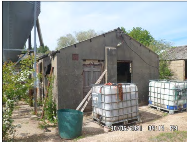
Photo 40: 'B14' in the southeast of 'Parcel 3' (southern gable end).
