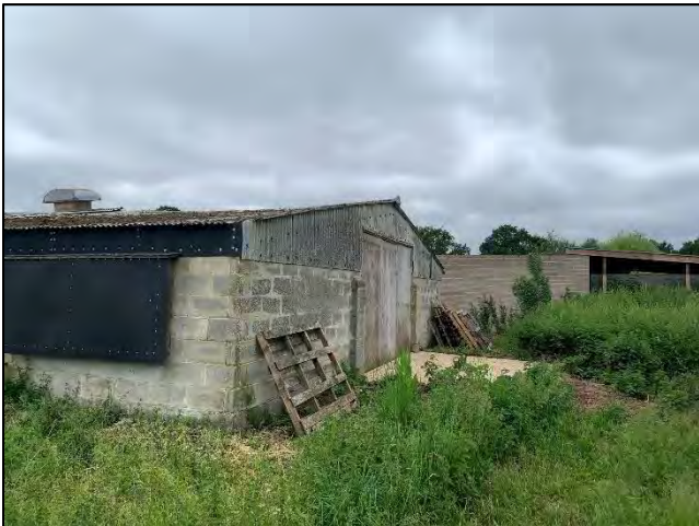
Photo 161: Northwest gable of 'B4' (northern section) viewed from the east.
