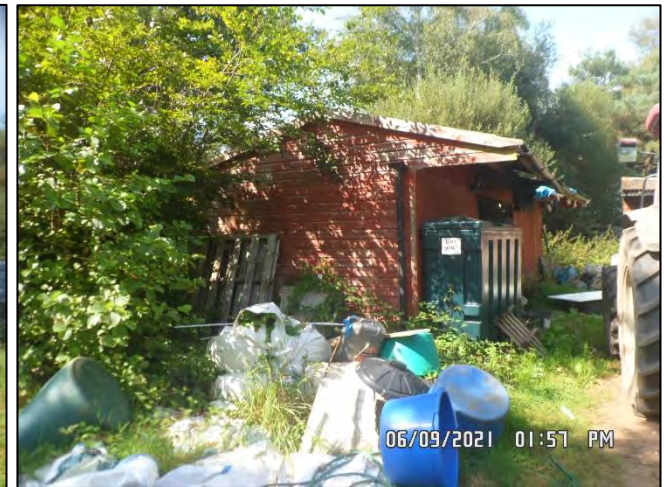
Photo 62: 'B6' in the centre of 'Parcel 4' viewed from the south.
