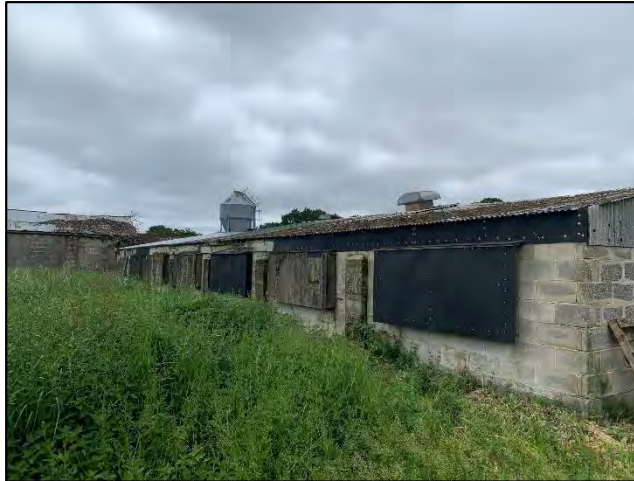
Photo 162: Northeast elevation of 'B4' (northern section of building).
