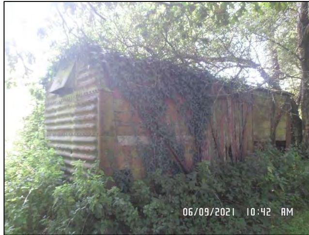
Photo 58: 'B8' in the northwest area of 'Parcel 4' viewed from the north.
