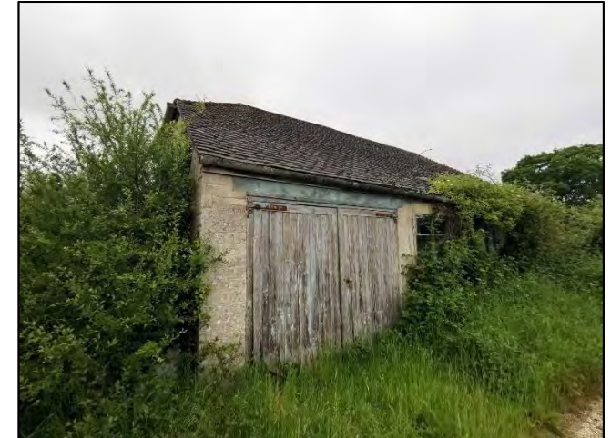
Photo 160: Northwest elevation of 'B2' showing double garage doors.
