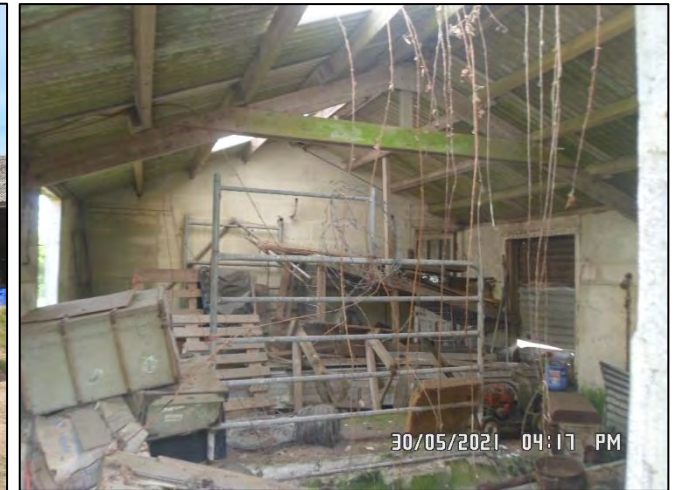
Photo 41: Internal of 'B14' in the southeast of 'Parcel 3'.
