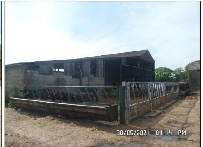
Photo 38: Eastern elevation of 'B12' with view from the southeast towards north/northwest.
