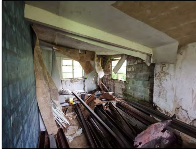
Photo 159: Internal of 'B2' (southwest side).
