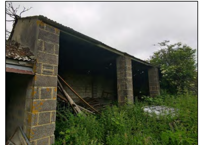
Photo 163: Southeast elevation of 'B4' and ruderal vegetation.
